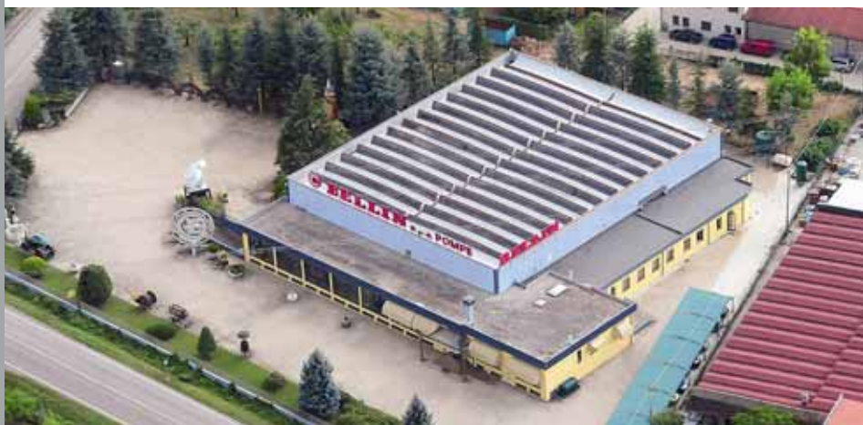
HEADQUARTERS - PRODUCTION UNIT 2
