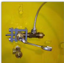
IVH-100-500 Isolation Valve Assemblies
